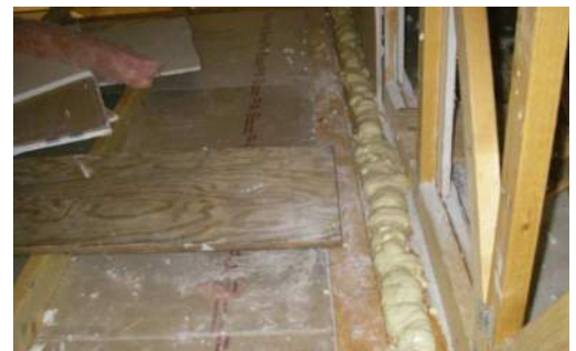
Spray foam installed over top plate joint.
