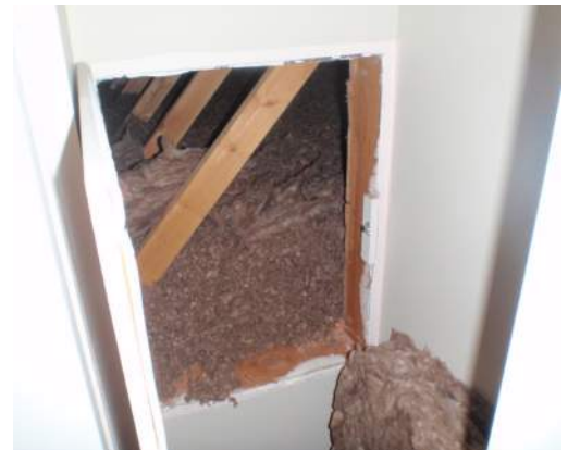
Access hatch at knee wall.
