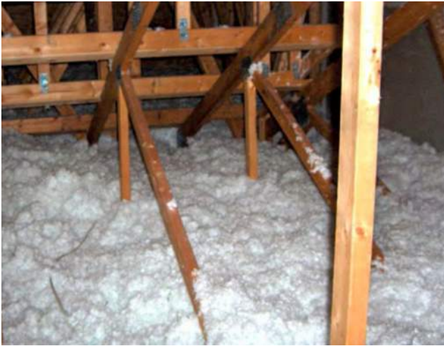
Blown-in attic insulation
