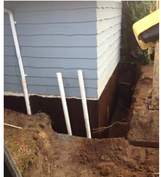
Adding exterior insulation to below-grade walls during foundation work is an effective way to increase the thermal performance of the wall.
