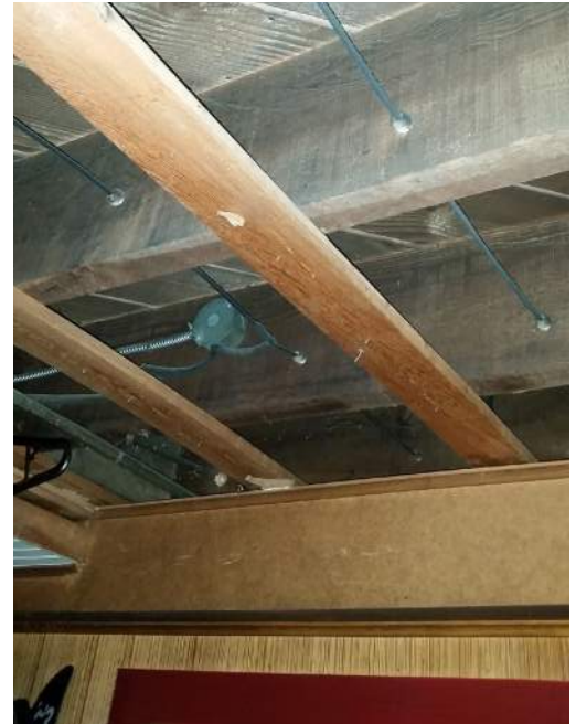
Non-insulated floor between a protected porch and a living space.
