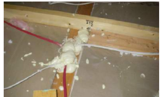
Top plate penetrations sealed with spray foam.
