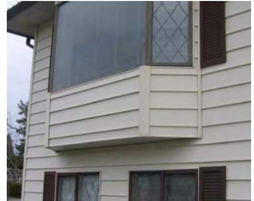
Overhanging floor under a bay window.
