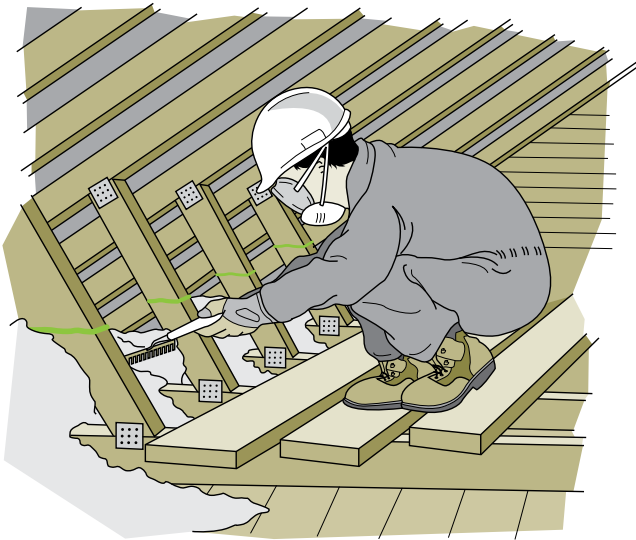
Figure 5-14 Installing loose-fill insulation
